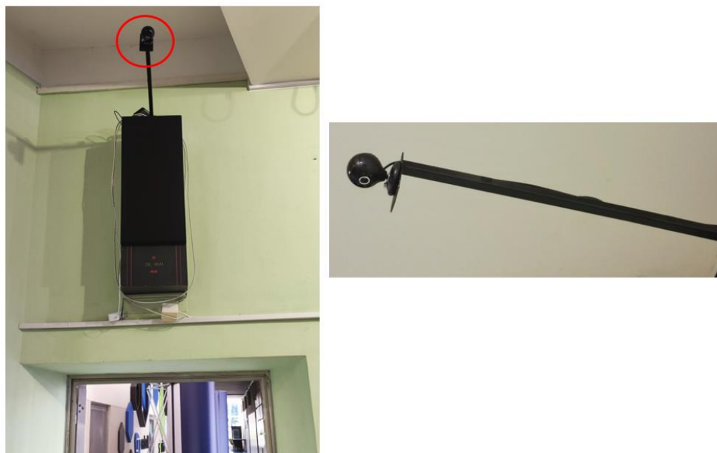
Figure 2: The mounted system above the entrance and the arm which holds the camera system
